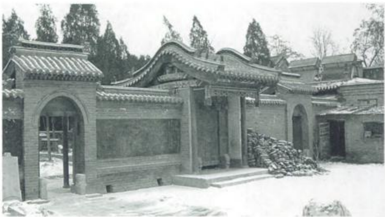
Fig. 1. Fuzhou Mosque in Hebei, constructed in the Yuan Dynasty.
